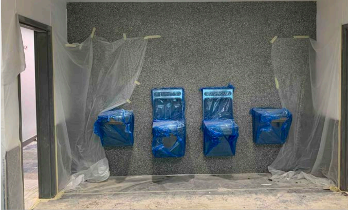
Drinking Fountain Accent Wall
