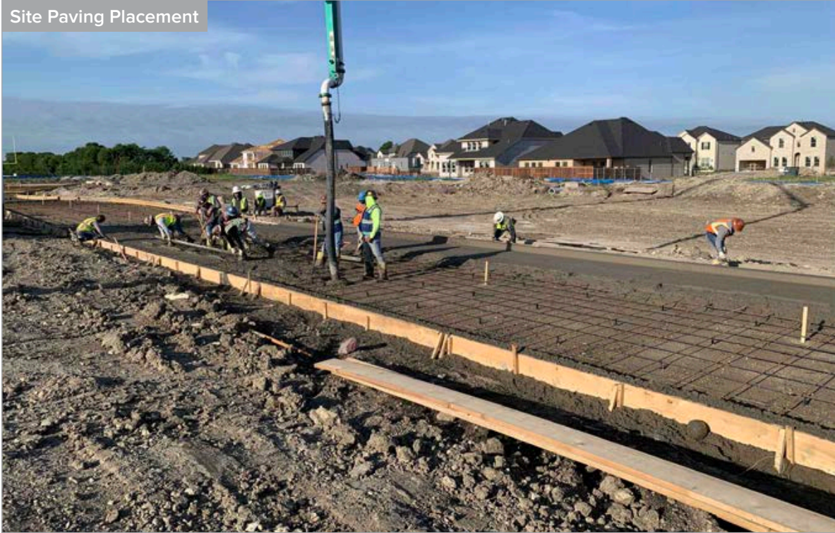
Site Paving Placement
